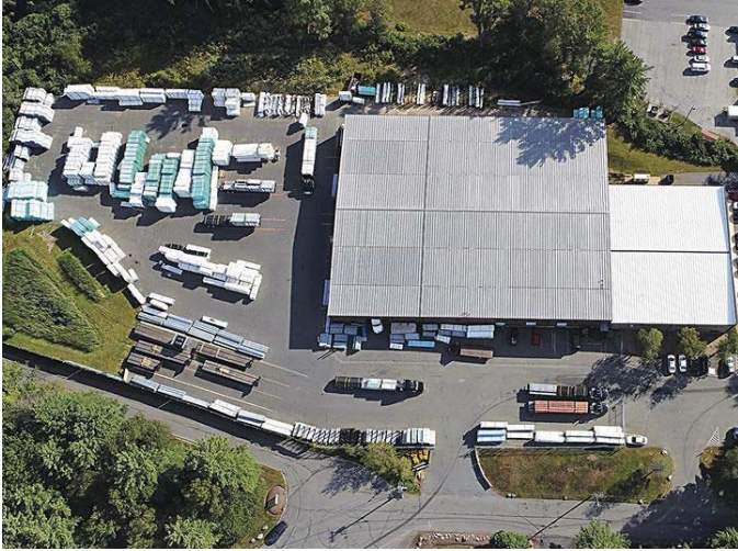
An aerial view of United Pipe's Ipswich, Mass., distribution center and corporate headquarters. The company recently opened its 12th DC in Stockton, Calif., and its 13th will go online next year in the Pacific Northwest. Photo courtesy of United Pipe & Steel.
